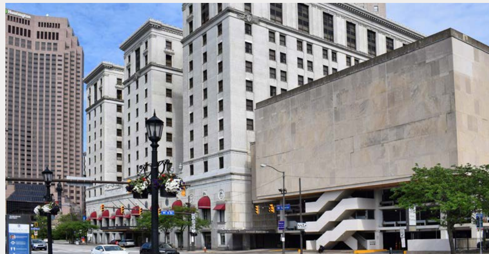
G - W 3rd & Superior facing southeast
