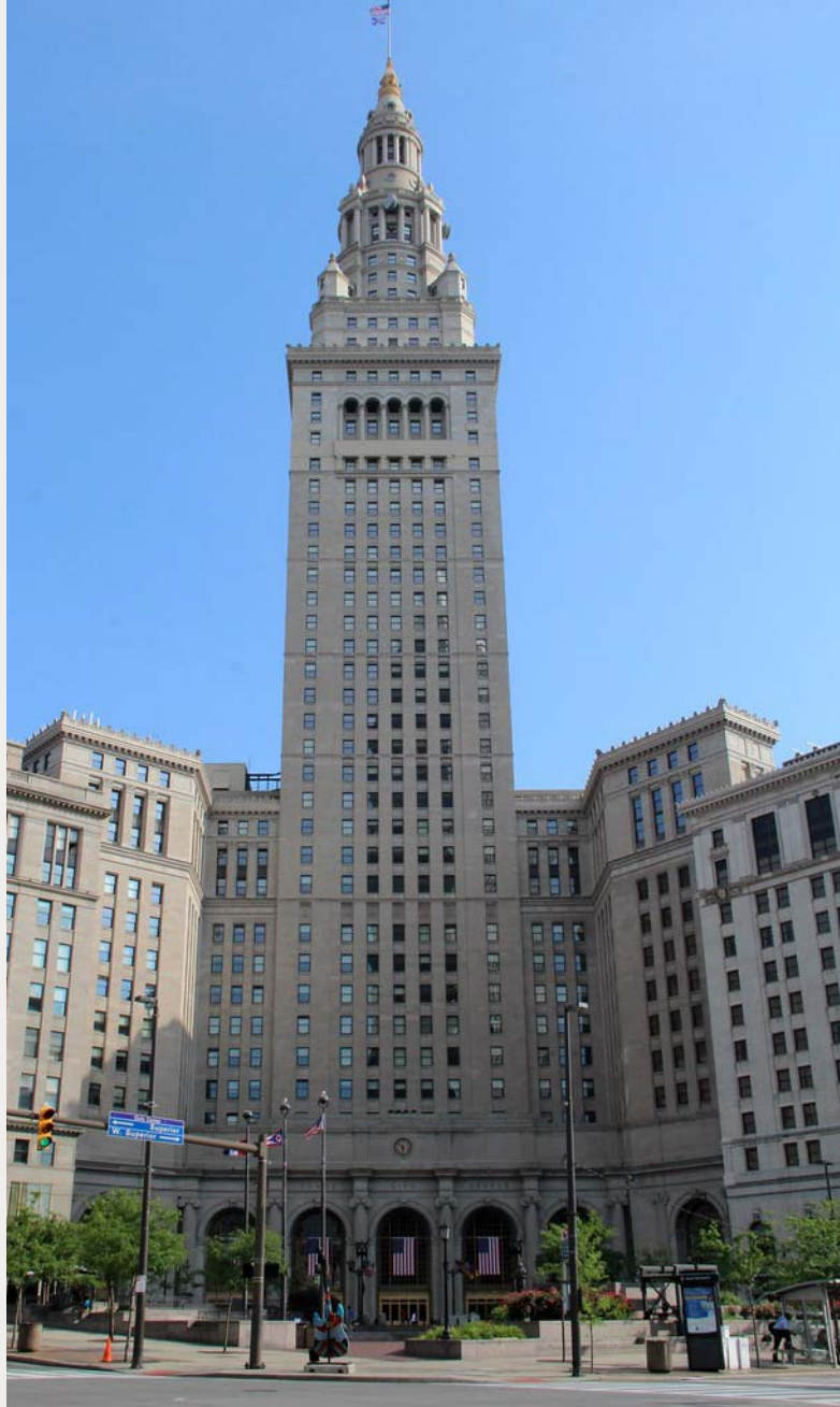
Terminal Tower & Renaissance Hotel
